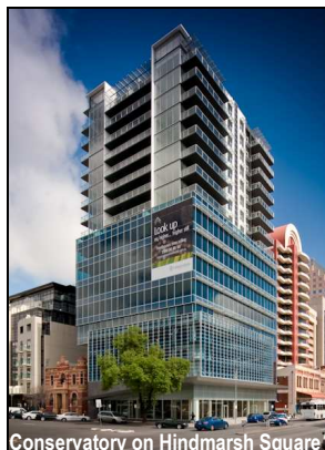
Conservatory on Hindmarsh Square
