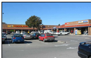
North Haven Shopping Centre 44-56 Osborne Road, North Haven
